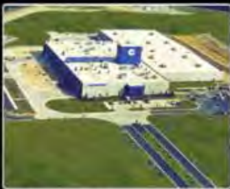
PAGELAND, SC Bronze Foundry and Manufacturing Plant
